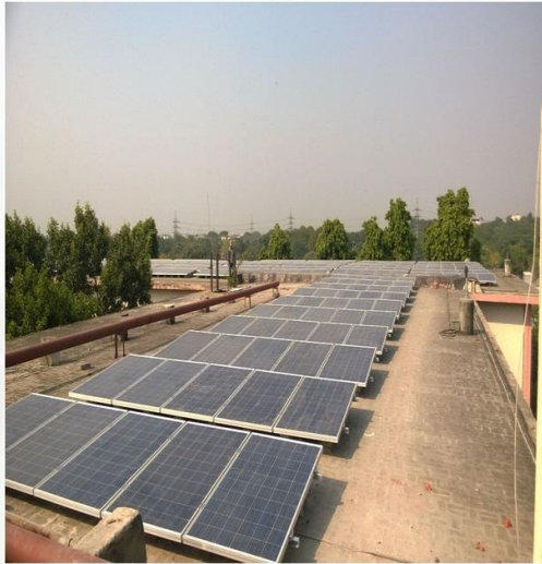
500 KWp Pushpa Bhawan New Delhi
