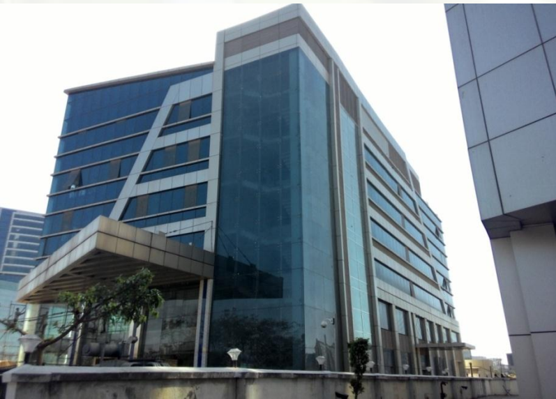
Regional Passport Office at Bandra Kurla Complex, Mumbai
