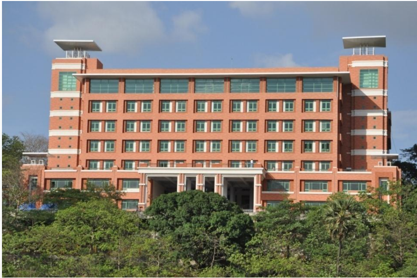
ADMN. & LIBRARY BUILDING FOR NITIE
