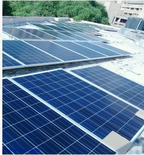
250 KWp at East Block R.K. Puram, New Delhi
