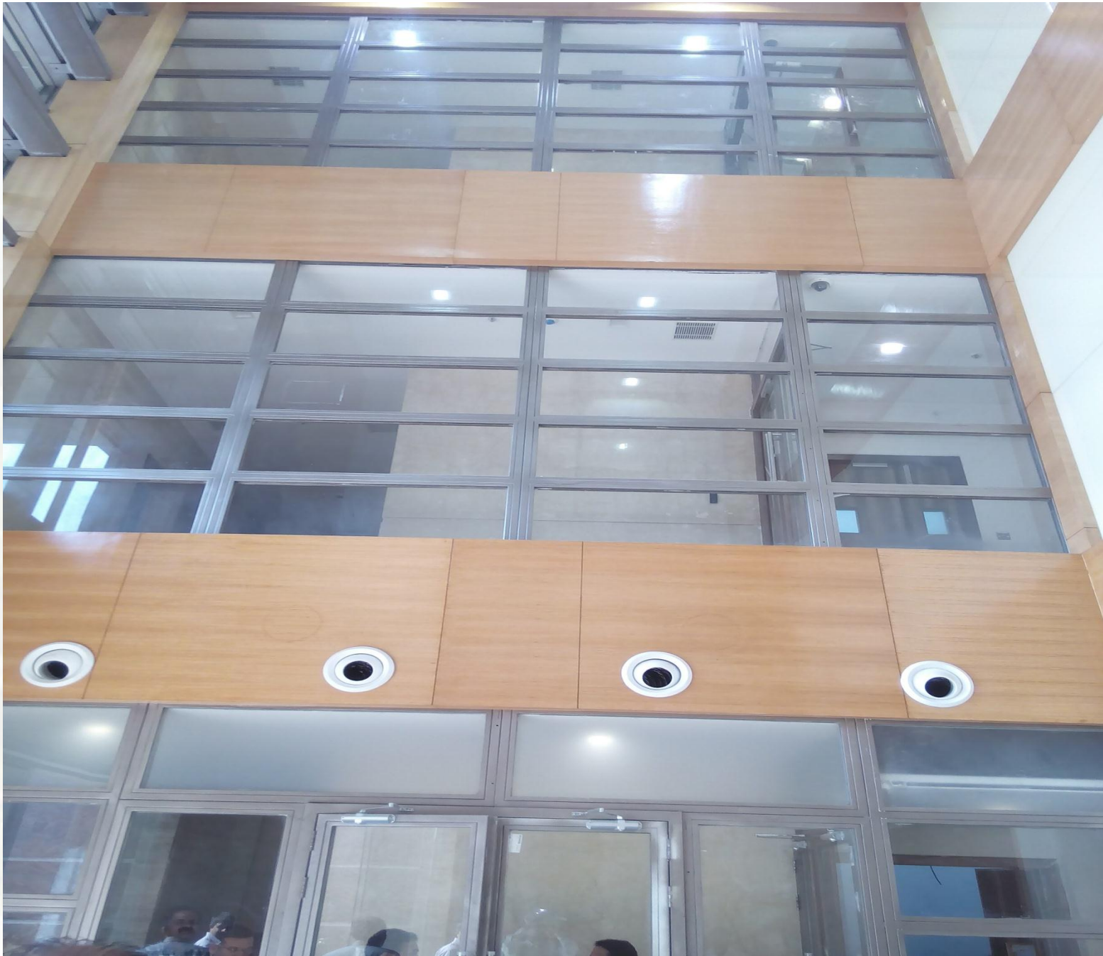
FIRE RATED DOOR AND GLASS PANELS IN LOBBY OF CBI BUILDING
