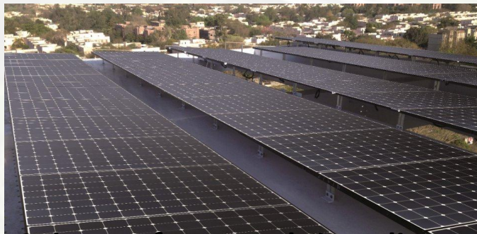
Solar Rooftop Panels in Indira Paryavaran Bhawan, New Delhi installed during construction
