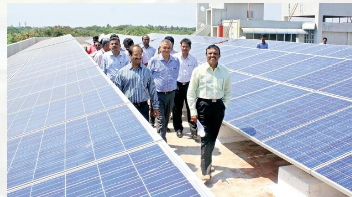
110 kWp at Chennai
